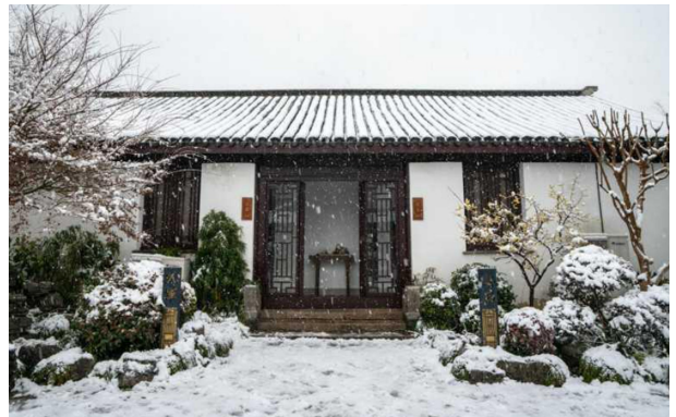
图 9 静乐院安石、右军包厢前踏雪寻梅雪景 Fig. 9 Anshi scenery in Jingleyuan Courtyard and snowy scenery of Taxue Xunmei in the front of wing-room
