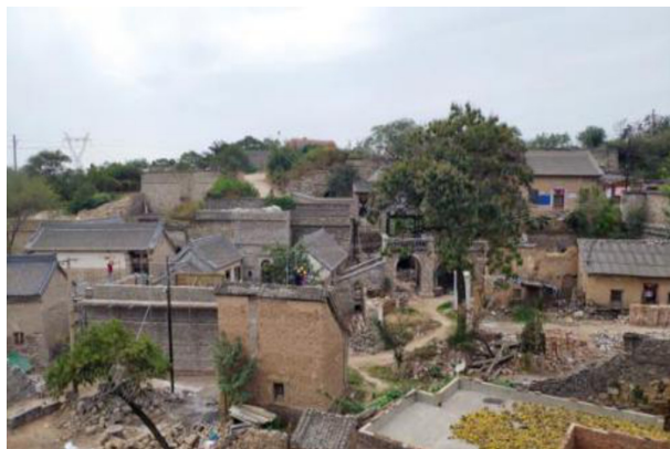
图 3 地形陡峭杂草满布 Fig. 3 Steep terrain and overgrown with weeds
