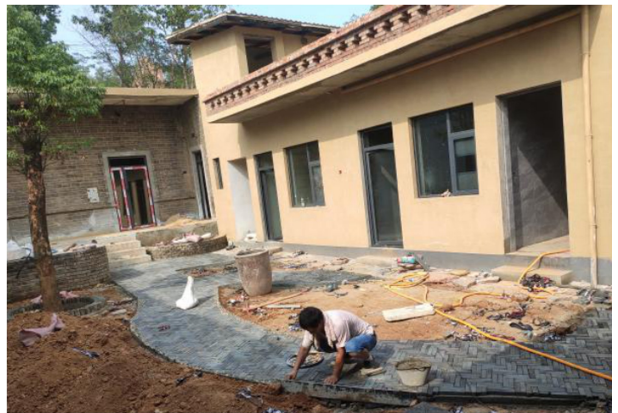
图 11 庭院外立面改造实景 Fig. 11 Real view of courtyard facade renovation
