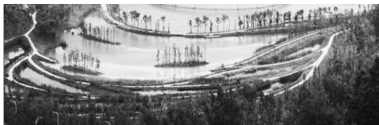
图 4 鱼塘生态改造效果 Fig.4 Effect of ecological renovation of fishpond
