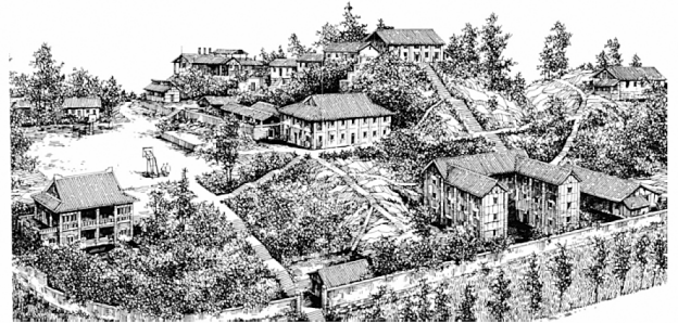
图 6 文德女子中学鸟瞰 Fig. 6 Aerial view of Wende Girls' High School
